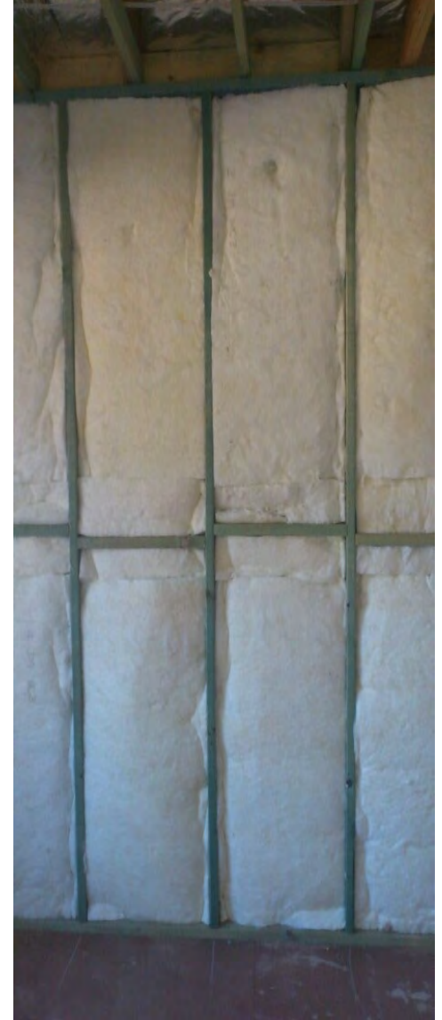
* Formaldehyde Free Glass Wool Insulation installed in walls for sound control
