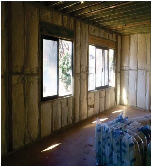
* Formaldehyde Free Glass Wool Insulation installed in residential walls
